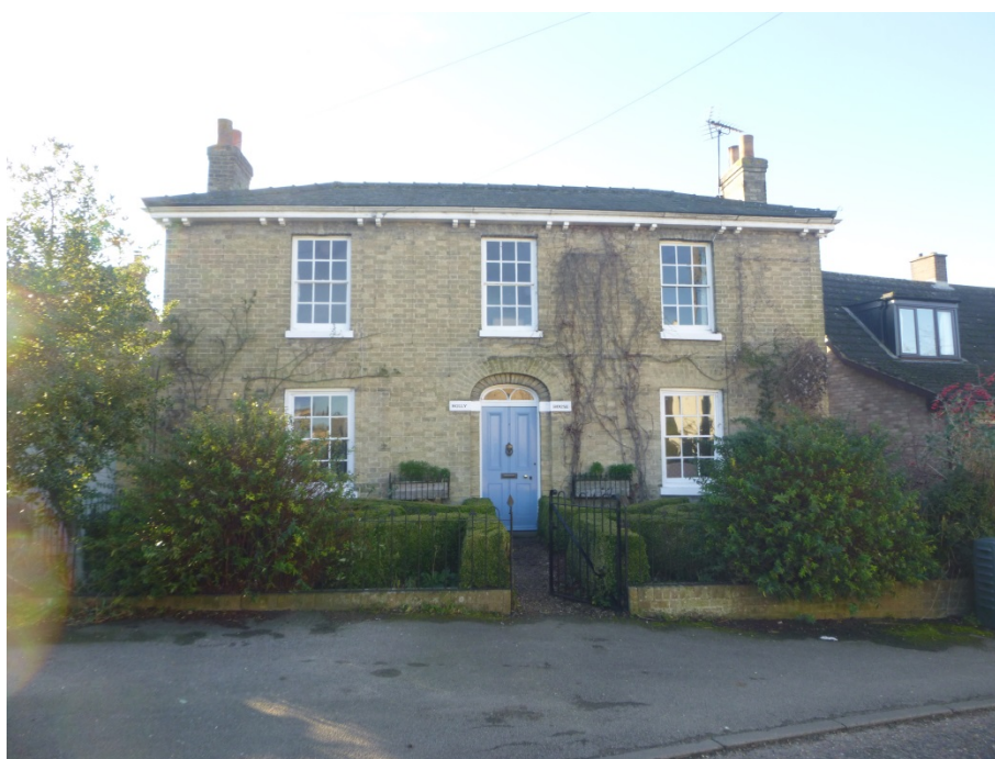
Photograph 5 -The photograph above illustrates distinctive residential architectural design typical of Waterbeach and South Cambridgeshire.
